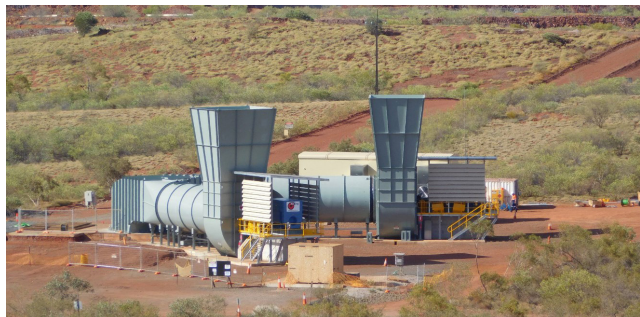
Figure 1. Full turnkey project for Newmont Tanami VR6 main ventilation fans with the installation of multiple monitoring systems.
