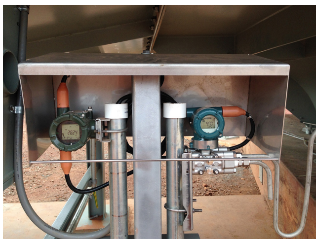
Figure 3. Newmont Tanami VR6 shaft collar pressure and air temperature monitors transmit real-time data with an automatic calibration.
